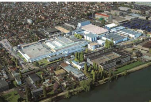
Sealants Europe facility in Bezons, France
